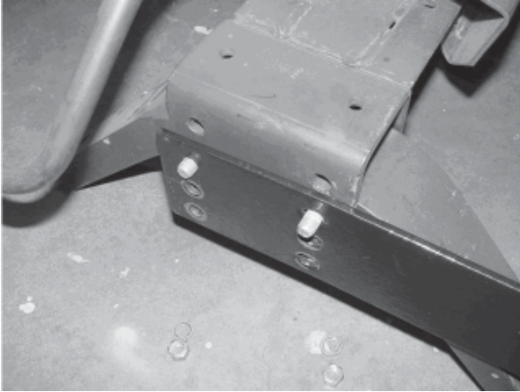
Figure 3-Left Side Plate installation
