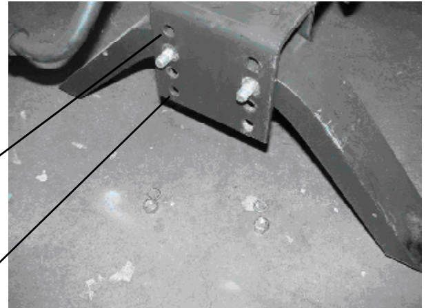
Figure 2-Left Side Frame Mounting Nuts removed
